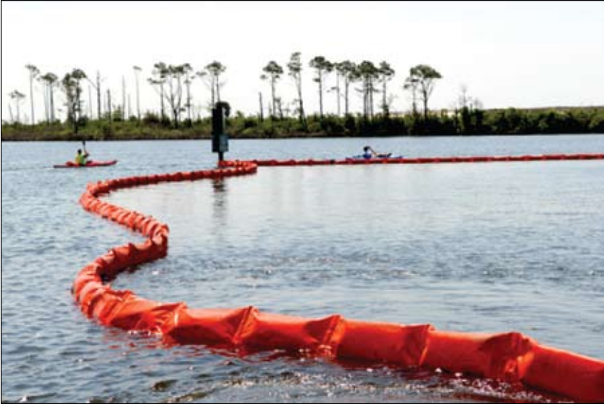
Figure 9: Containment boom during Deepwater Horizon response, Pensacola, Florida.
